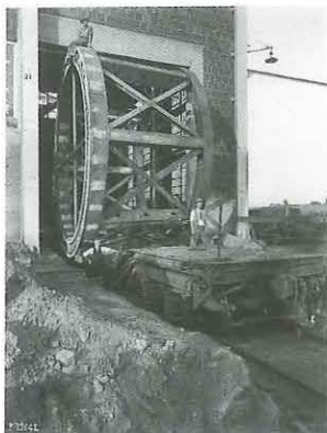
Right: After it was shipped across country from Corning, New York, as crowds lined the tracks to watch, the giant mirror spent nine years (and occupied 180,000 man hours) being ground and polished in Caltech's optical shop (later reincarnated as the synchrotron building). About 30 tons of abrasives were used to grind it down from 20 tons of Pyrex to less than 15 tons.
